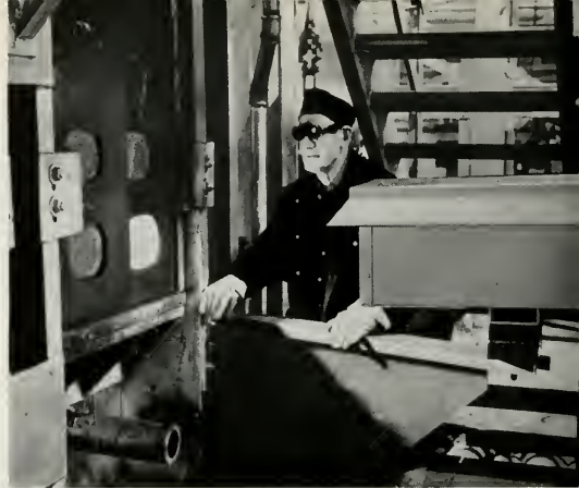
peers into a steel mill reheating furnace . . .
